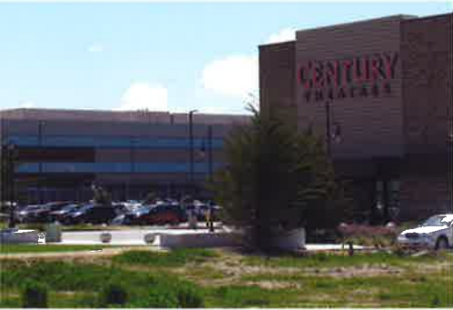
Newly constructed Cinemark movie theatre and the VA/DoD Veterans Clinic.
