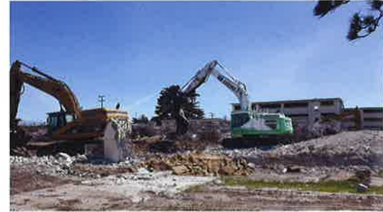
Building removal at CSUMB.
